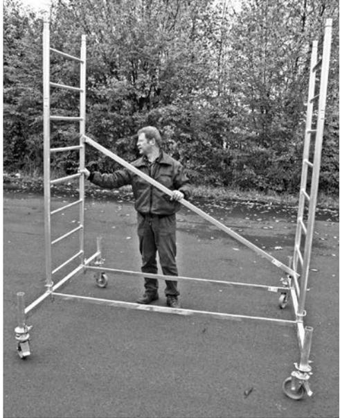
Attach the second diagonal to the fifth rung of the vertical frame to the first rung on the other side (see picture), so that it is at angles to the first brace. Secure it with the safety set.
