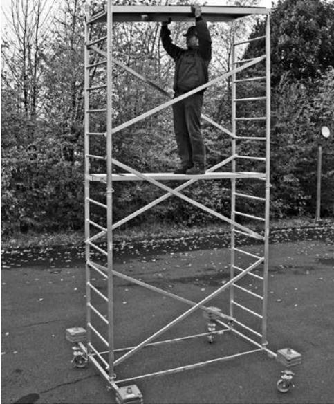
Attach the board to the top rungs of the vertical frames. Secure it by tightening the previously mounted safety sets.
