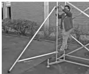
The picture shows an attached outrigger.
