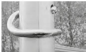
All plug-type connections must be secured with scaffold clips.
