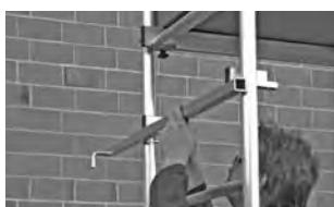
The picture shows how to adjust a stabilizing set.
