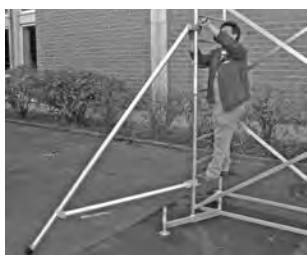
The picture shows an attached outrigger.
